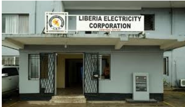
Figure I.3. Liberia Electricity Corporation, Waterside Monrovia
