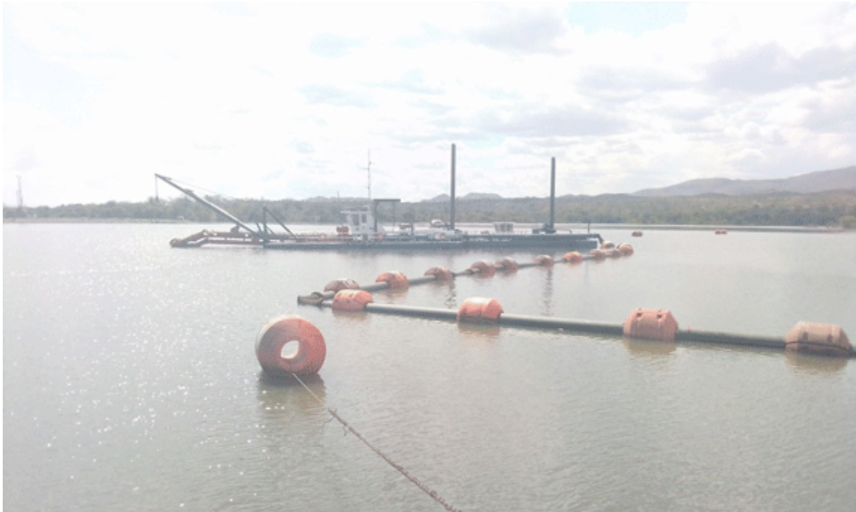
Figure IV.9. Dredge at Kapichira connected to floating pipeline
