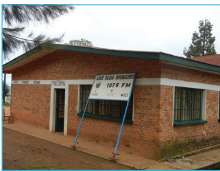
Headquarters of the Ishingiro radio station.
