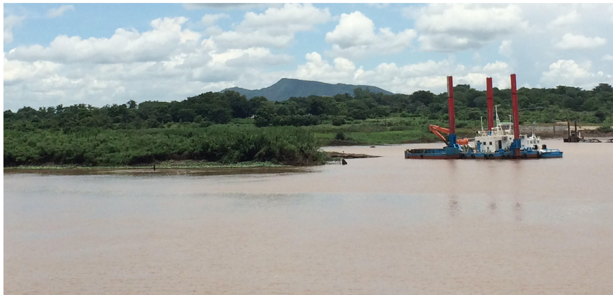
Figure IV.6. Island of sediment and weeds and old dredging equipment at Nkula head pond
