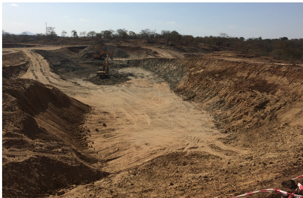
Figure IV.9. Sediment disposal area under construction: Kapichira power station, November 2018
