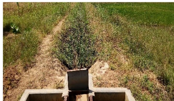
Clogged tertiary canal
