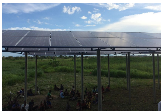
Solar panels providing energy to the FISD irrigation scheme
