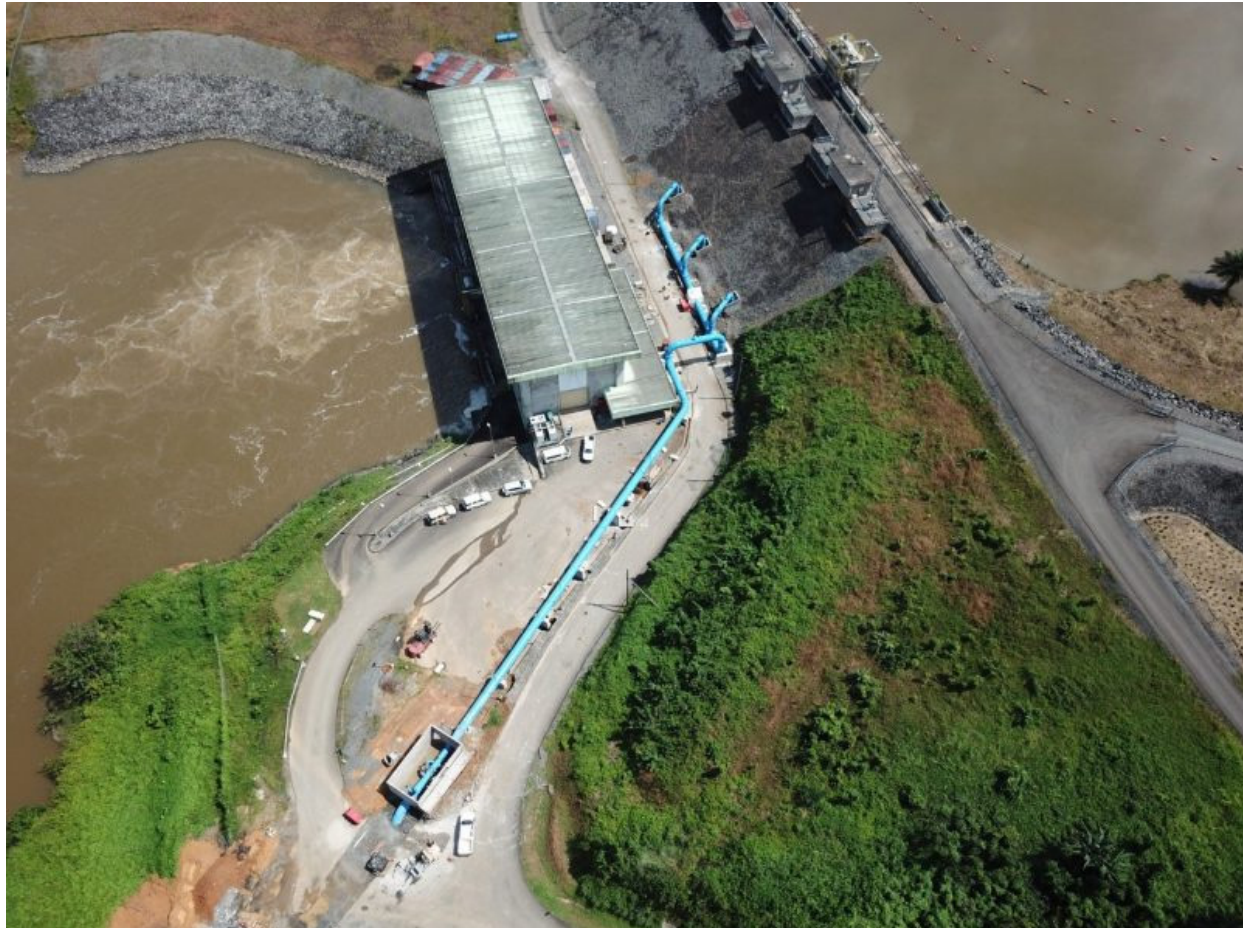
Figure III.3. Finished pipeline segment
