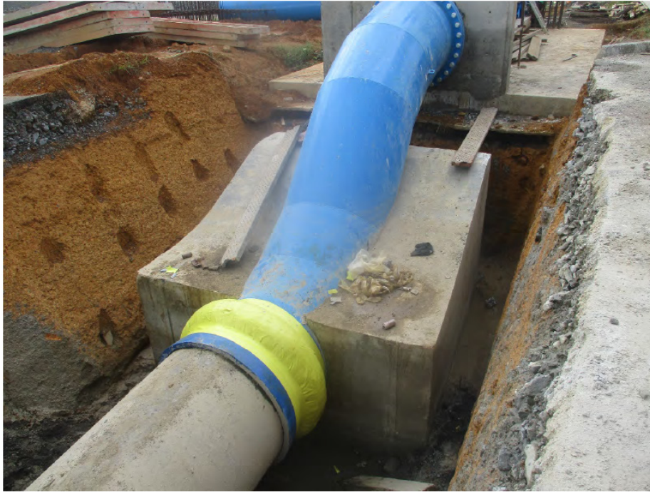
Figure 2. Photos from the construction of the pipeline
