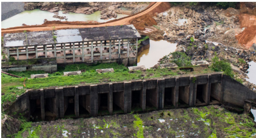
Figure I.2. MCHPP before rehabilitation
