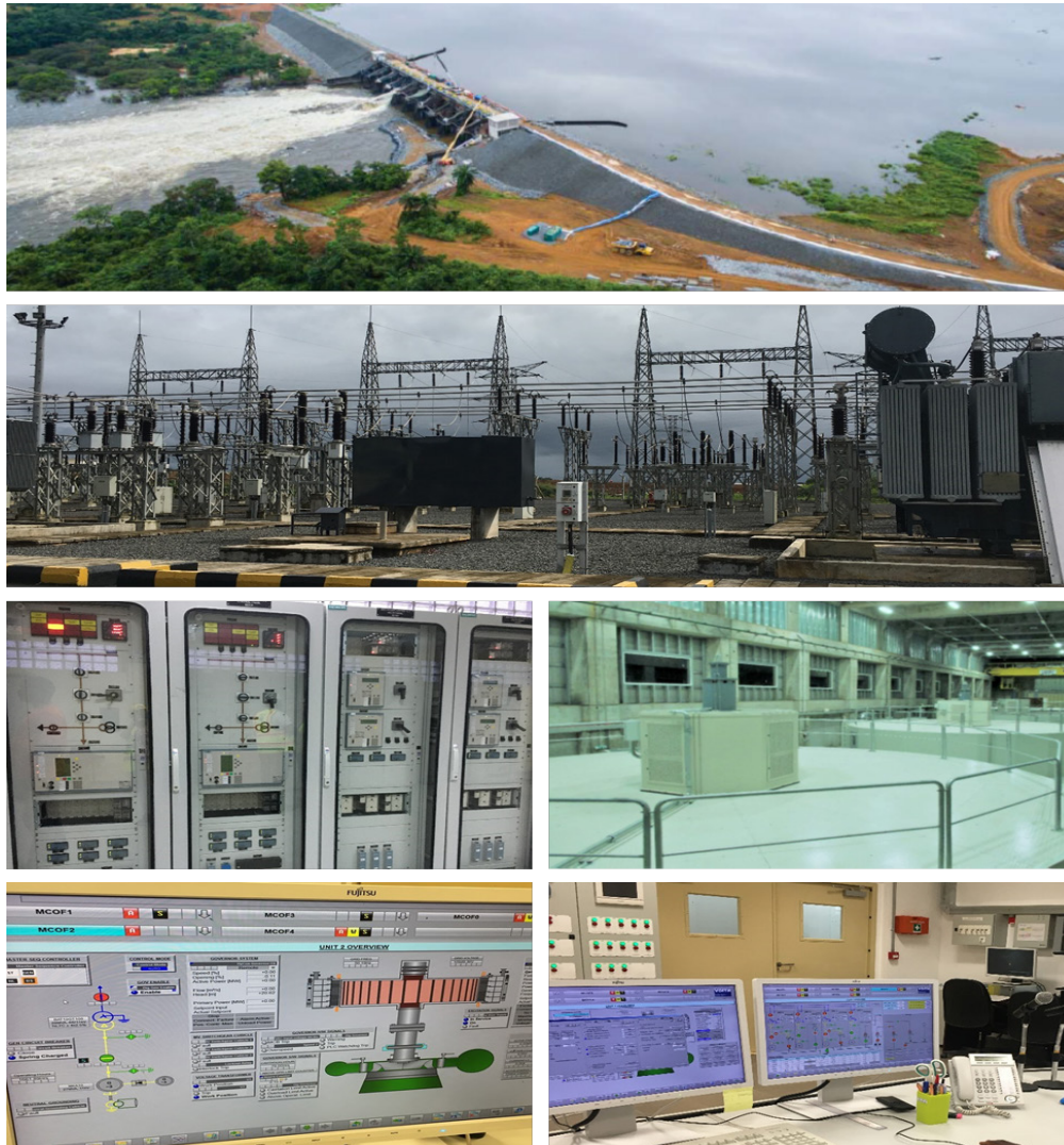
Figure V.3. MCHPP aerial view
