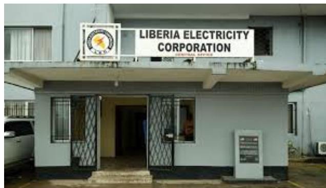
Figure V.2. LEC Headquarters at Waterside
